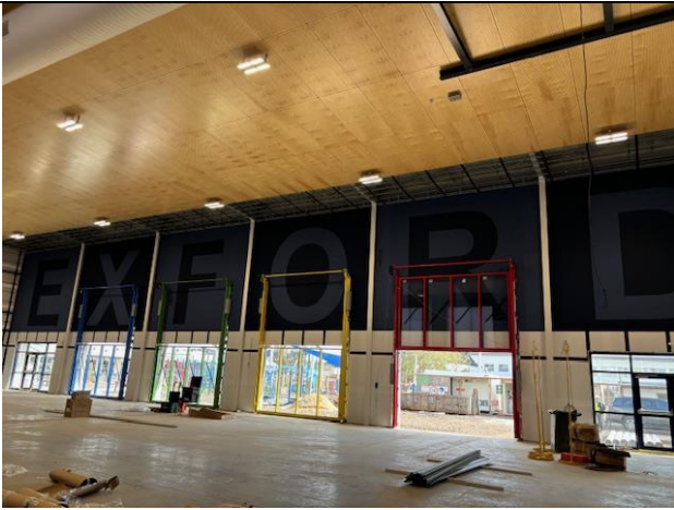
If you look closely, you can see the 'EXFORD' lettering above the hydraulic lift-up doors that will open up the side of the Gym onto the playground.
